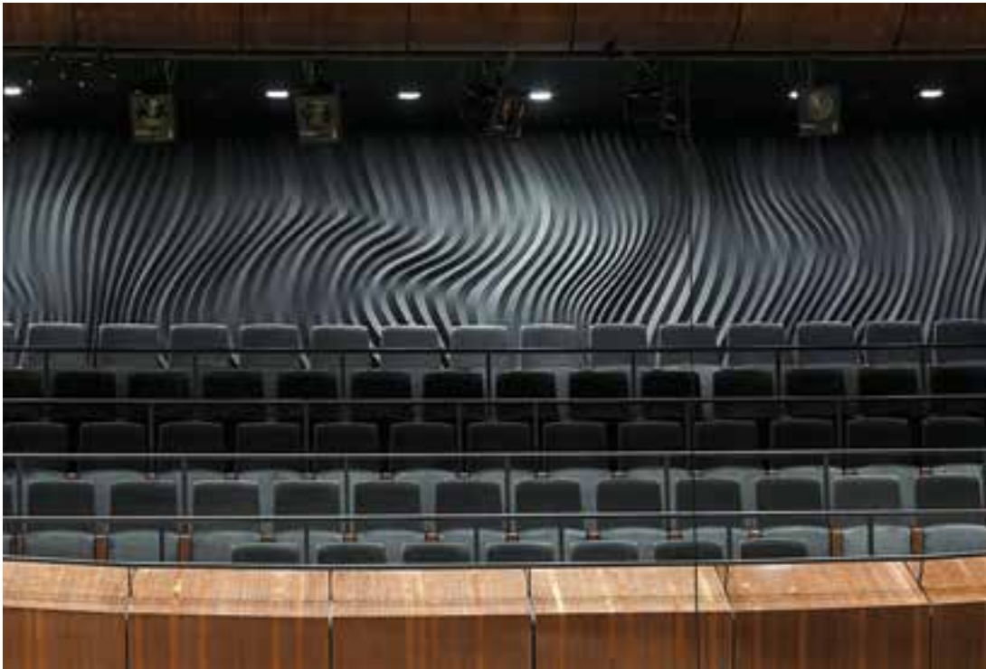
THE ARCHITECTS DECIDED ON GIVING THE CONCRETE A STRUCTURE. THE PATTERN WAS DESIGNED DIGITALLY AND PRODUCED WITH RECKLI FORMLINERS.
